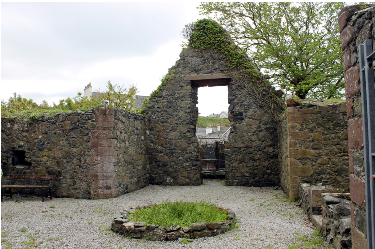
13. Internal view of south transept with doorway and window. Aumbry in east transept to left.
