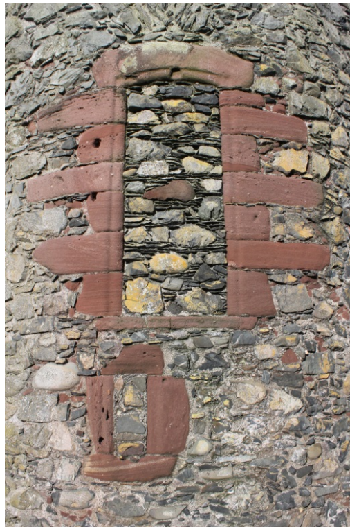
24. Detail of windows on east face of tower.
