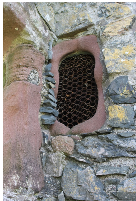
22. Tower window overlain by north-west corner wall of west transept
