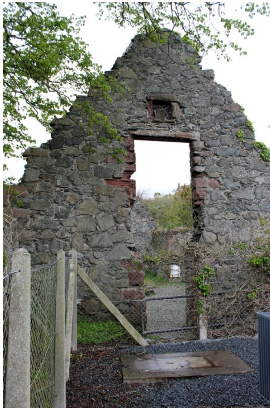
9. South gable with window & doorway.
