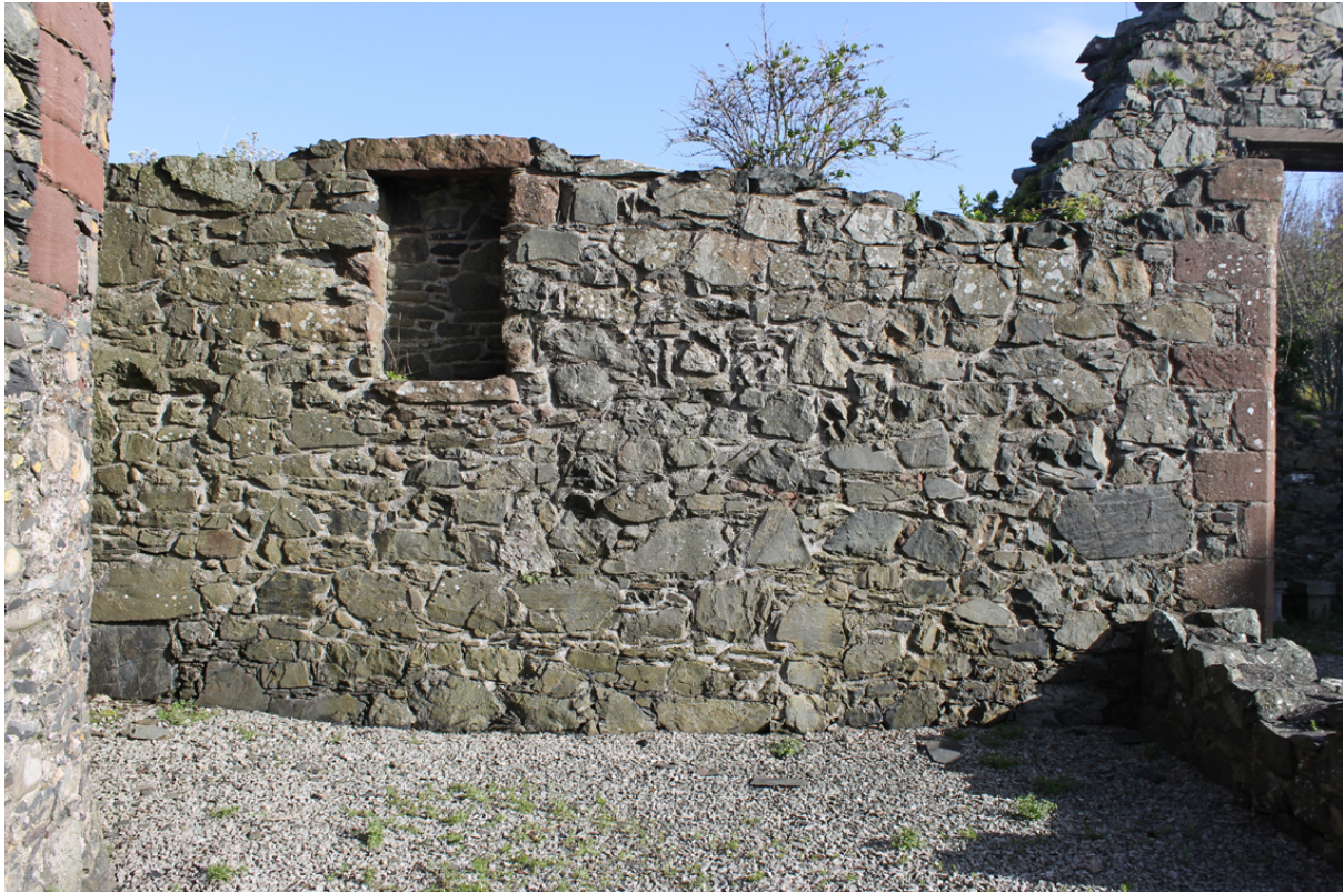
16. North wall of west transept with blocked window.
