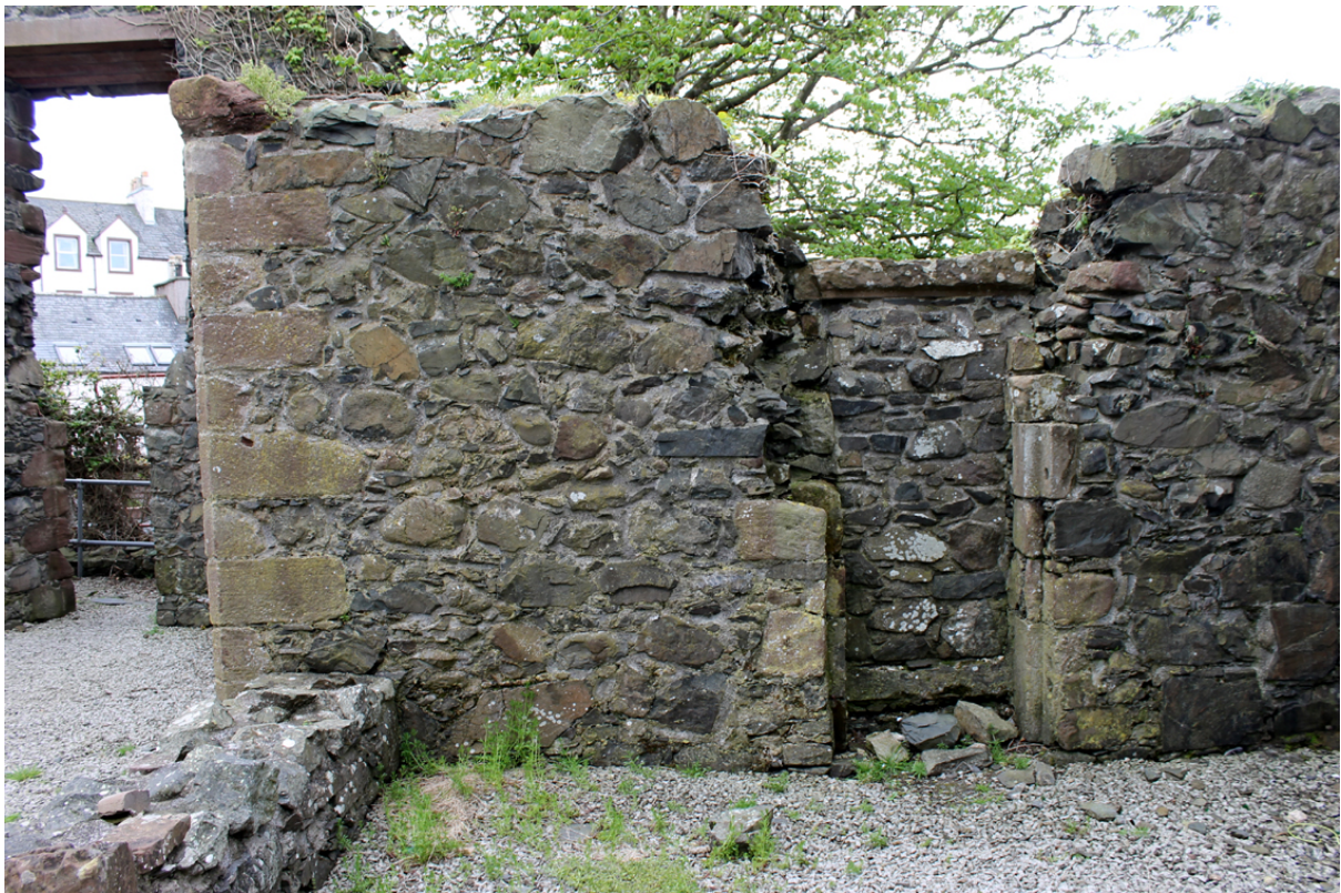
17. South wall of west transept with blocked doorway.
