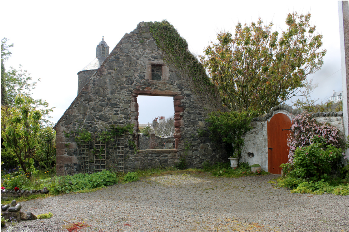
12. East transept with window and heraldic recess.
