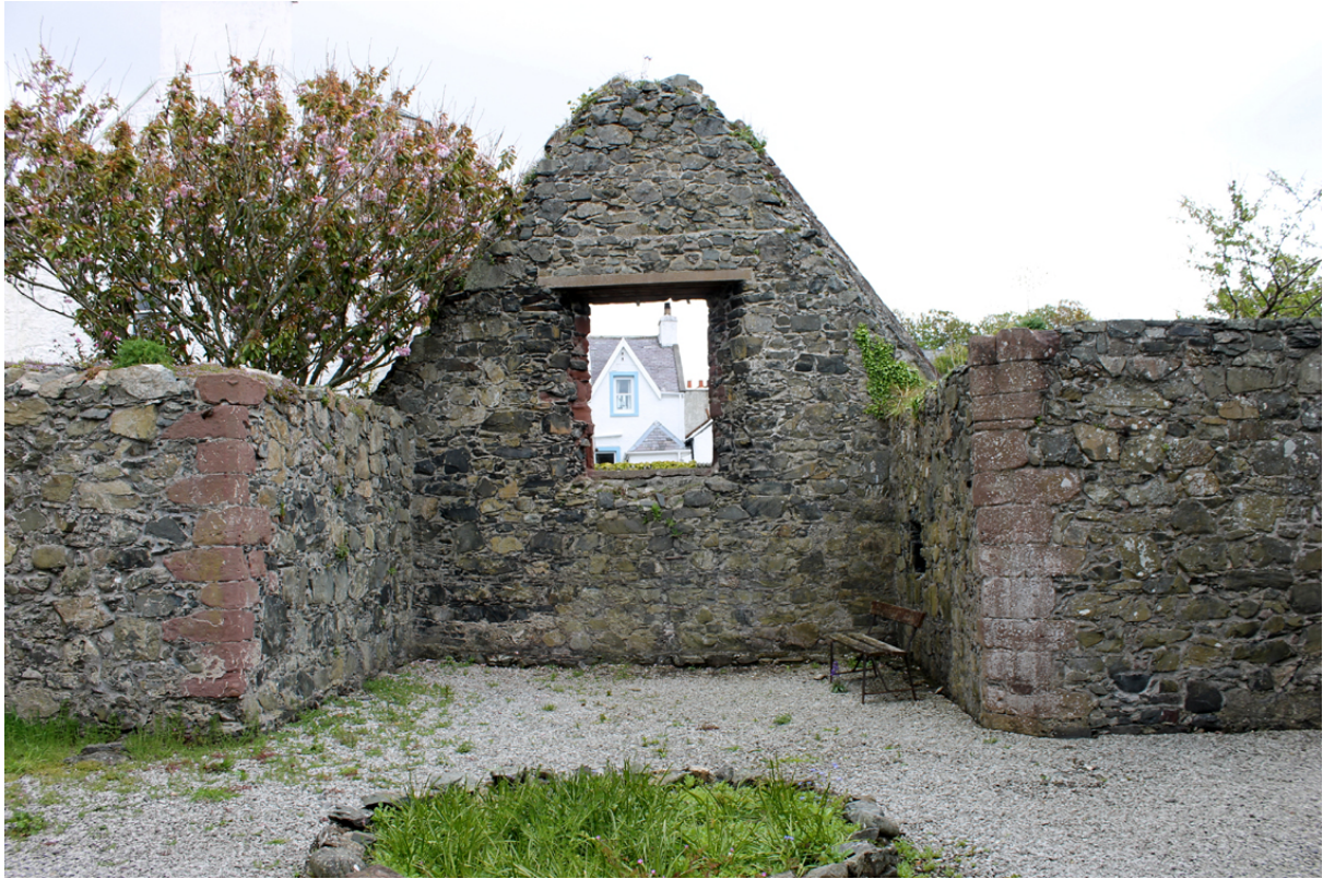
14. Internal view of east transept.
