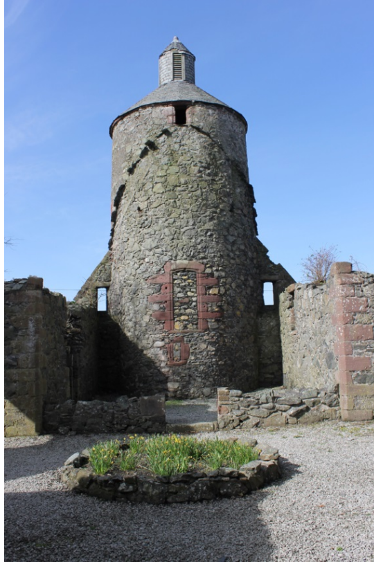
23. View of tower from east showing former roof line and west transept cross wall.
