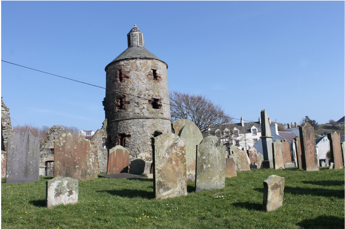
18. View of tower from north-west.
